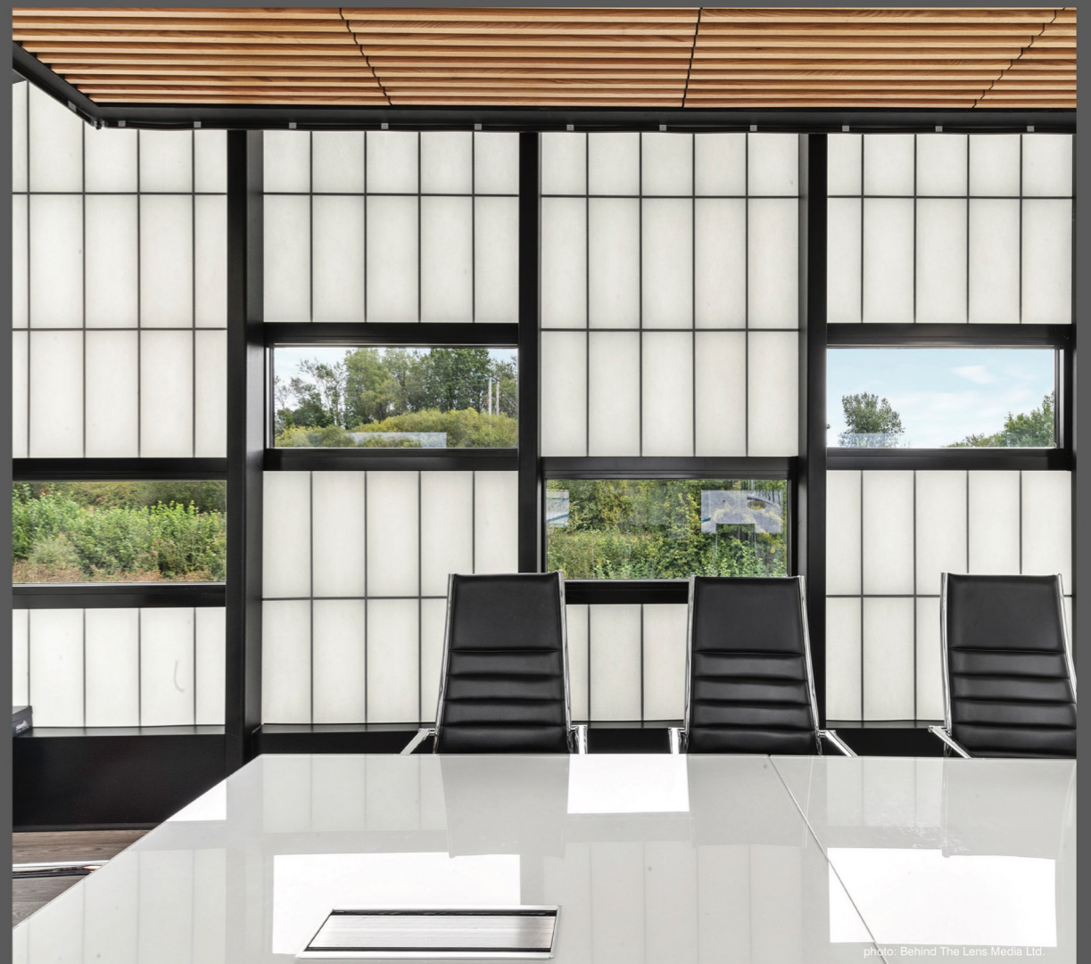
Frank's Ice Cream | Wales, UK | Sauro Architectural | Kalwall TIGU in curtain wall by others
